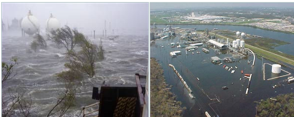
Figure 2: Storm Surge and Flooding Post-Katrina at Petrochemical Facility
